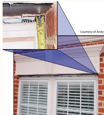
Vertical Differential Movement at a window head, four story building constructed in 2003
