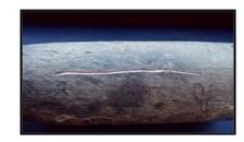
Lead service lines are generally a dull gray color and are very soft. You can identify them easily by carefully scratching with a key. If the pipe is made of lead, the area you've scratched will turn a bright silver color.
