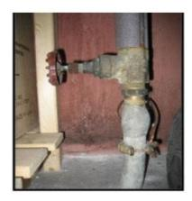
Lead service lines can be connected to the residential plumbing using solder and have a characteristic solder "bulb" at the end, a compression fitting, or other connector made of galvanized iron or brass/bronze.
