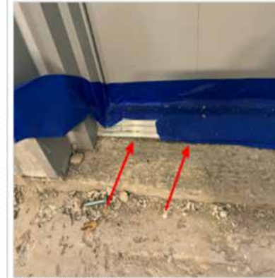
Leakage at door threshold
