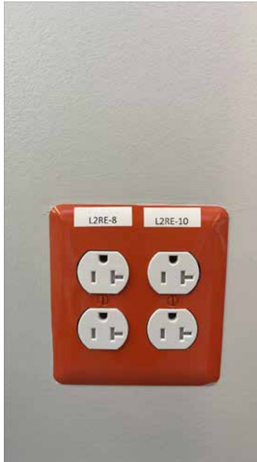
Occupancy-controlled receptacle stays on despite 30 min lack of motion
