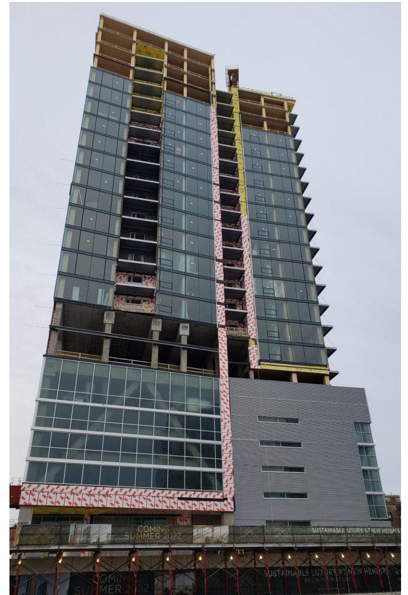
Level 26 (Roof) Topped Out (December 2021)
