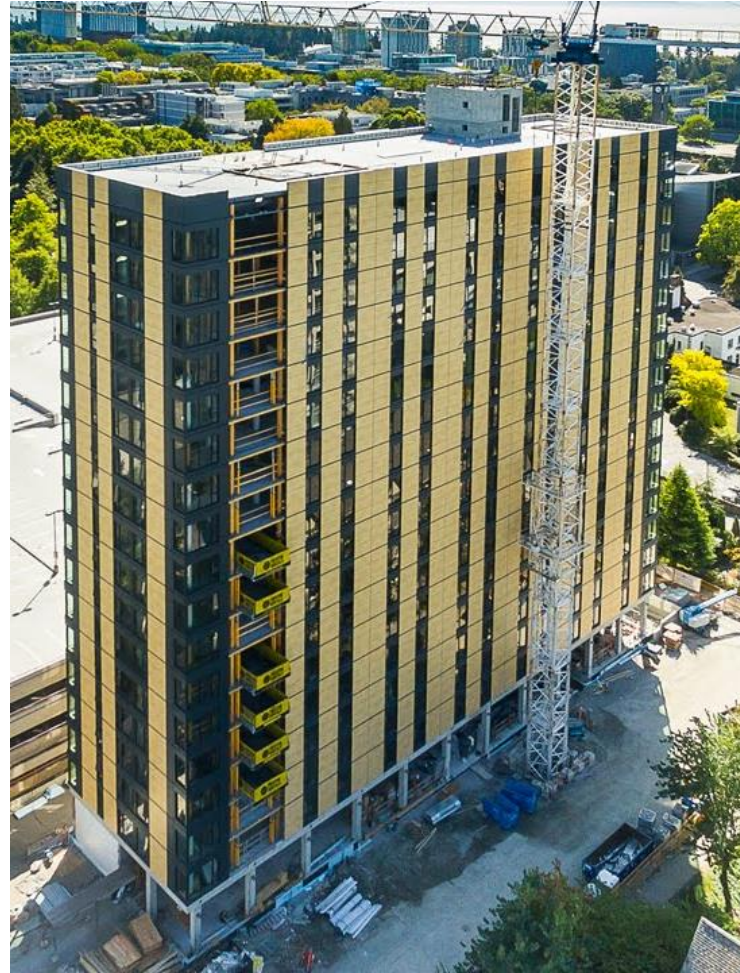
Brock Commons, Vancouver, Canada (18 stories)
