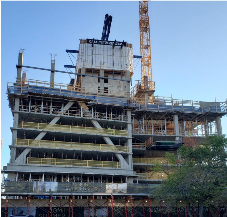
Start of Timber Construction (June 2021)
