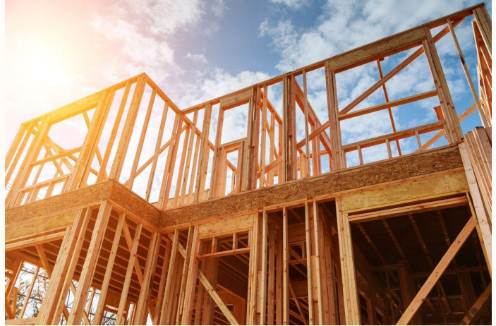
Tolerances for Wood Framing?
