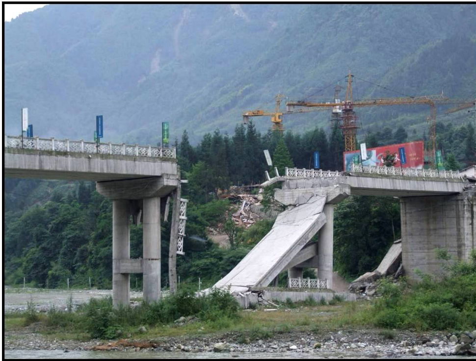
Figure 4-11 – Bridge with fallen span (China)
