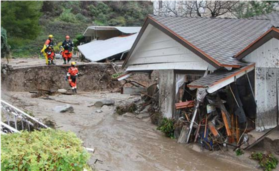
Figure 3-22 Debris flow damage to house
