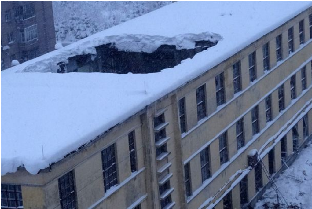
Figure 3-34 - Roof collapse due to snow
