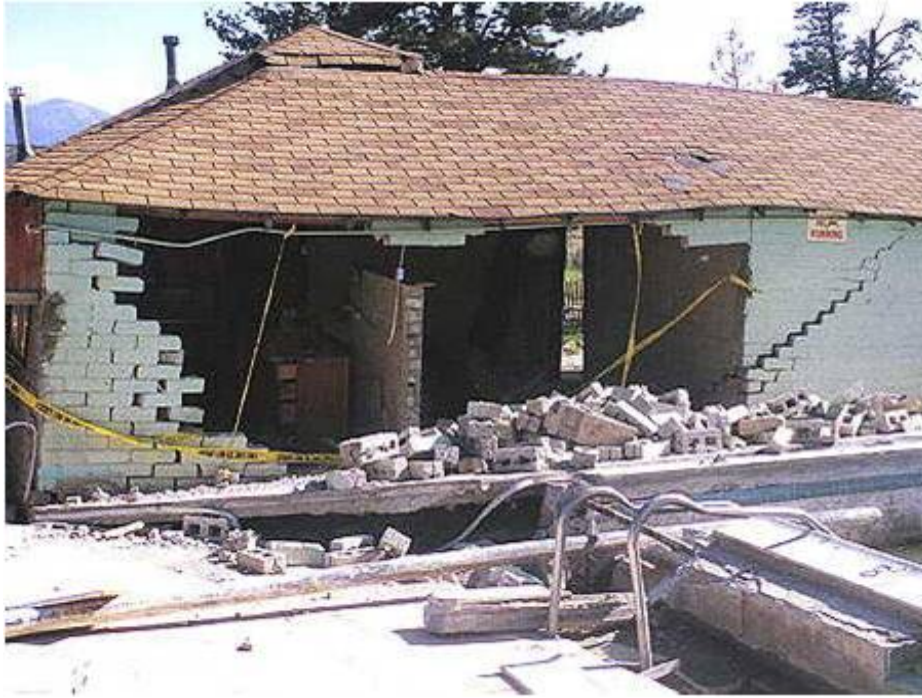
Figure 2-18 – Uplifted pool and damaged URM building, 1992 Big Bear Earthquake
