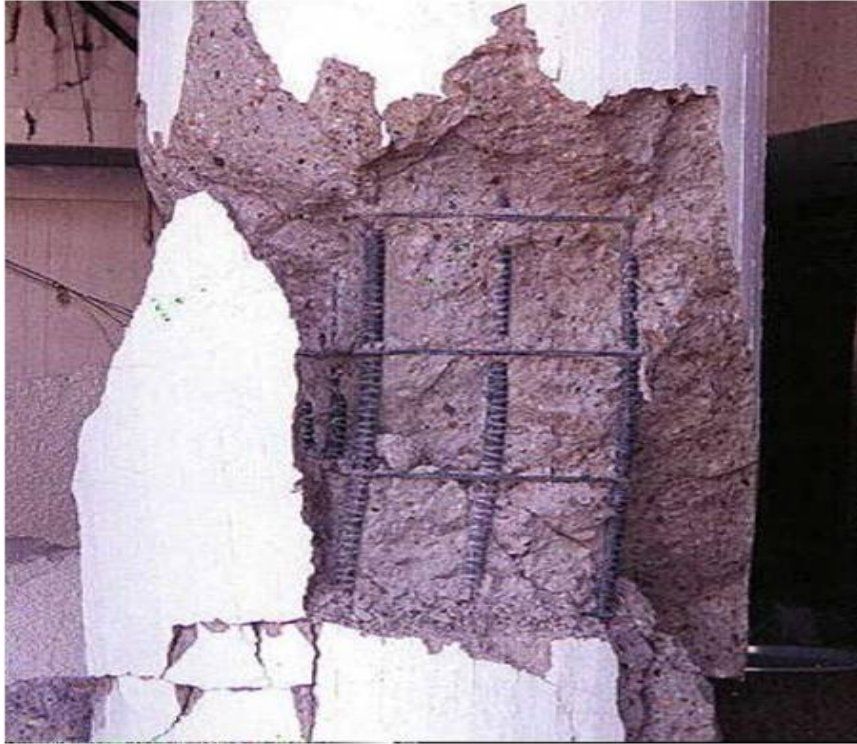
Figure 2-20 – Detail of damaged column showing P-delta effect
