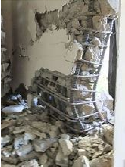
Figure 2-7 – Non-ductile concrete wall failure
