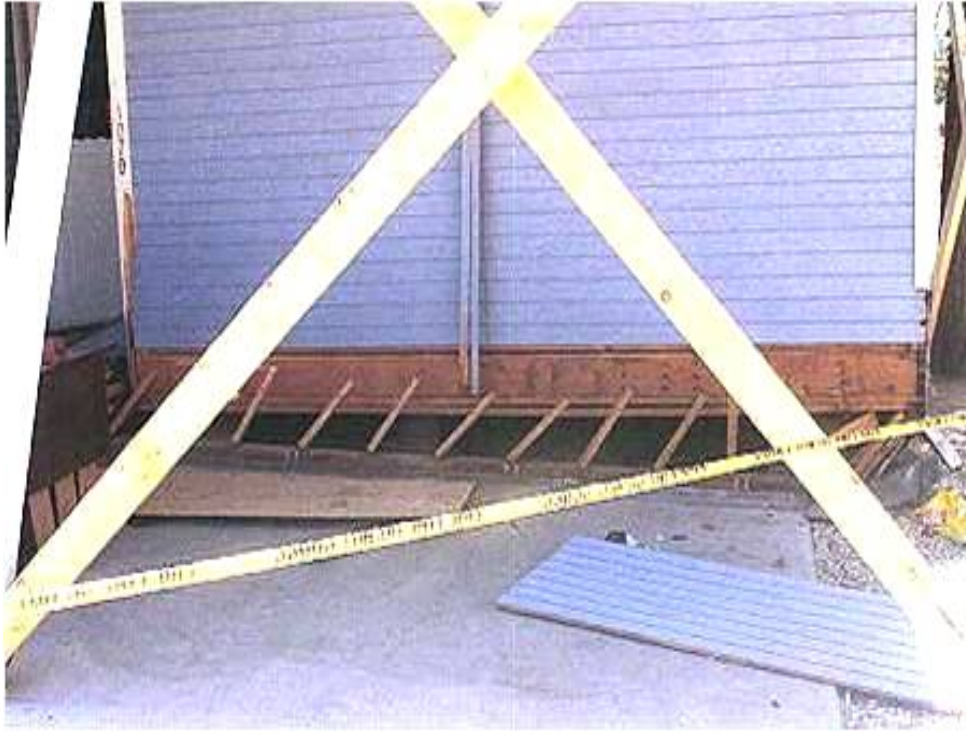
Figure 6-20 – House with cripple wall failure, 1992 Big Bear Earthquake
