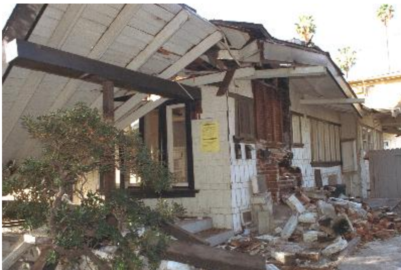
Figure 2-15 – Yellow tagged home, 1994 Northridge Earthquake
