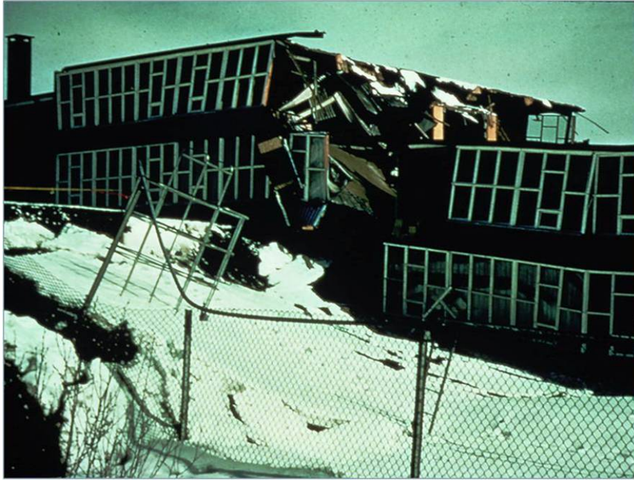
Figure 2-9 – Ground scarp through building
