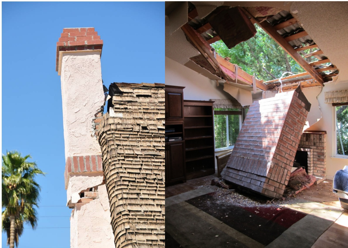
Figure 2-12 – Damaged chimneys
