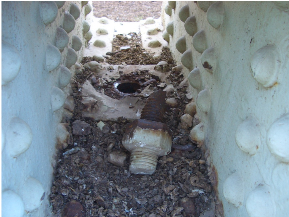
Figure 2-25 – Damage to water tower concrete footing
