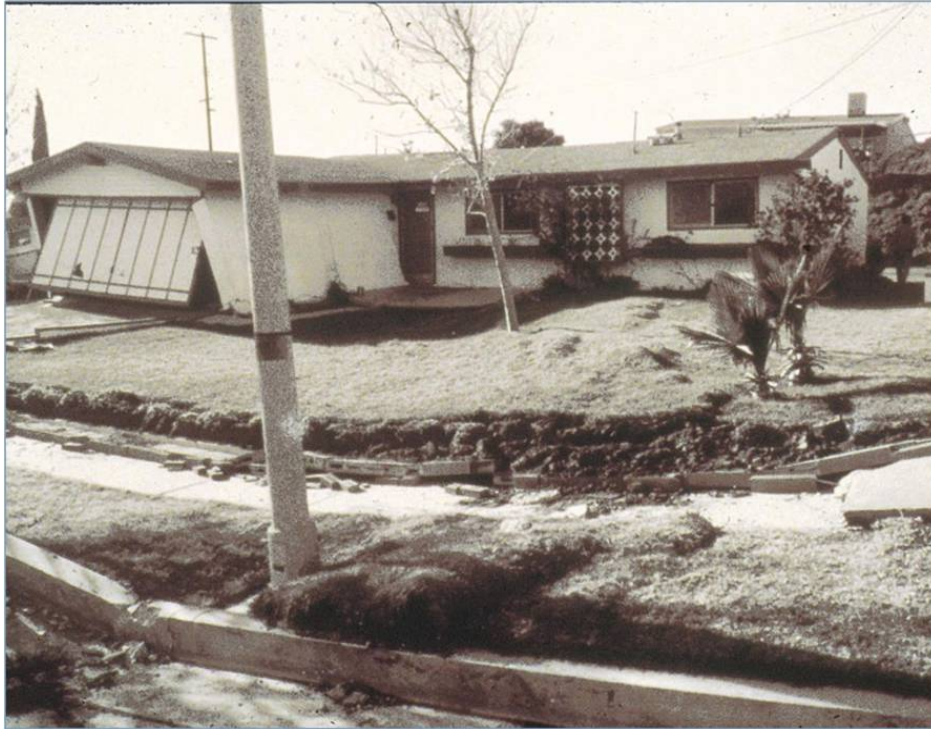
Figure 4-2 – Surface rupture, 1971 Sylmar Earthquake
