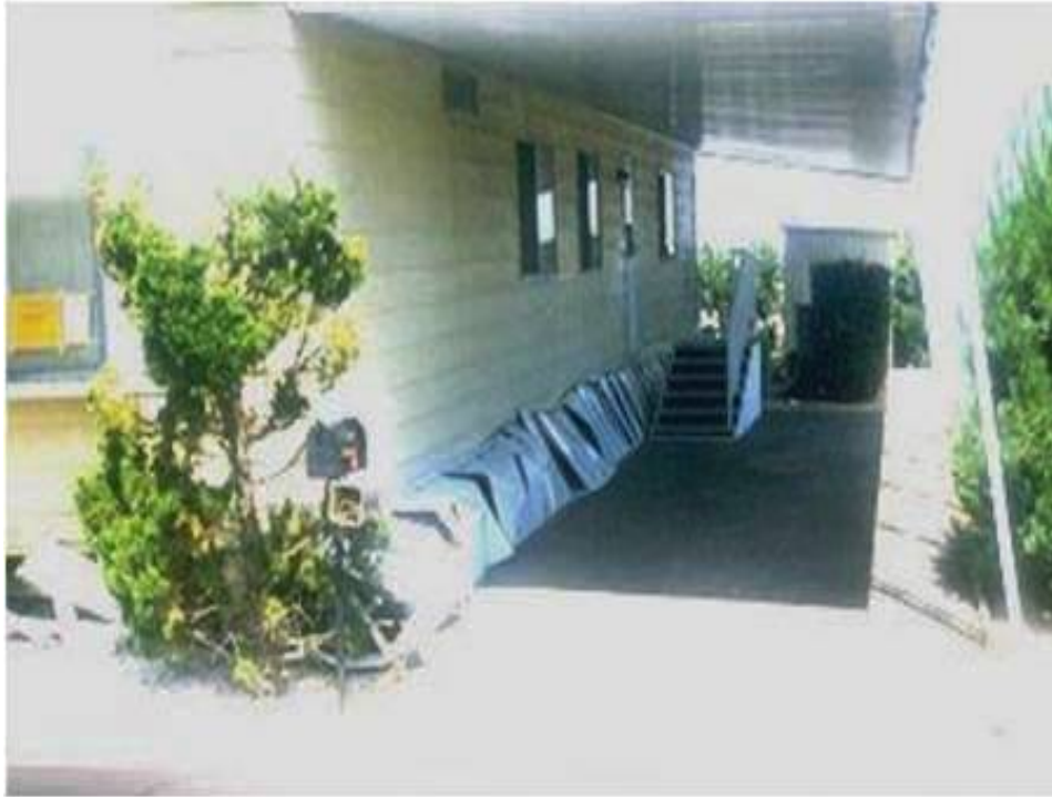
Figure 6-3 – Mobile home partially fallen, 1992 Landers/Big Bear Earthquakes
