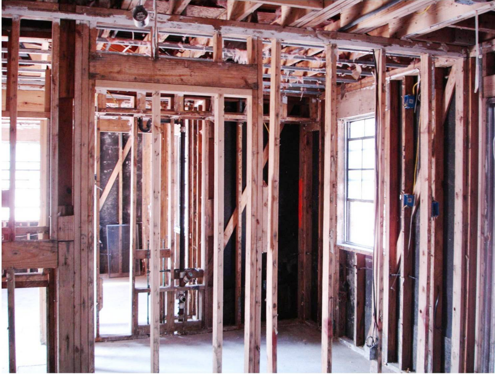
Figure 3-11 – Wood frame structure under cleanup, 2005 Hurricane Katrina
