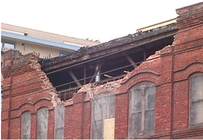
Figure 2-16 – Unreinforced masonry wall failure, 2001 Nisqually Earthquake.
