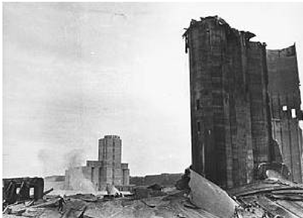
Figure 3-25 – Explosion – damaged granary
