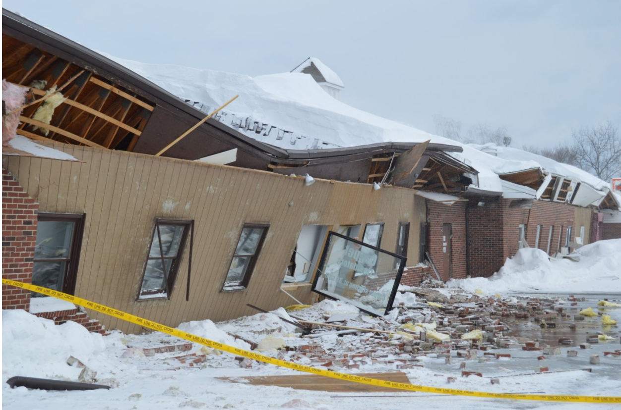
Figure 3-36 - Snow-caused roof and structure collapse in Massachusetts.
