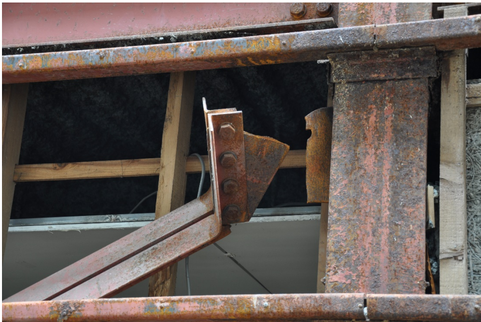
Figure 2-20 – Detail of damaged column showing P-delta effect
