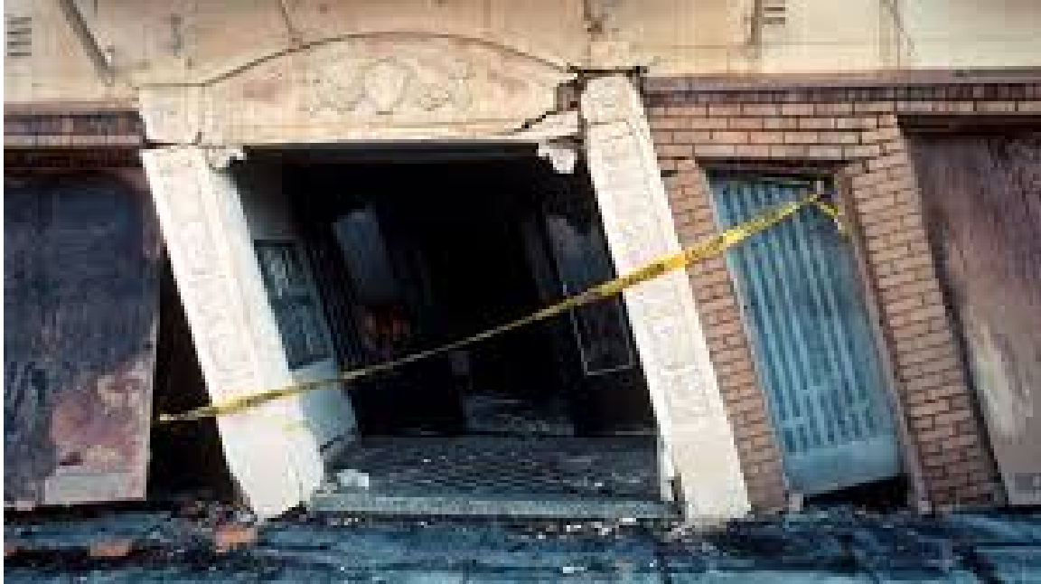
Figure 2-11 – Soft story racking damage.
