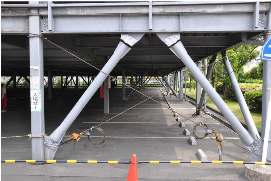
Figure 2-23 – Failed gusset plates on lateral bracing
