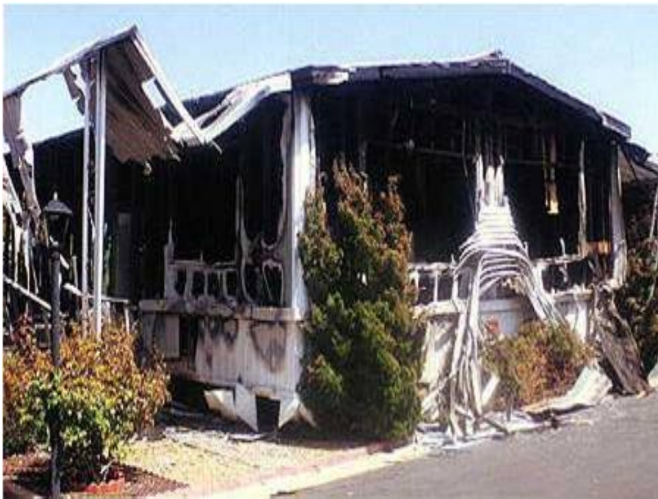
Figure 6-3 – Mobile home partially fallen, 1992 Landers/Big Bear Earthquakes
