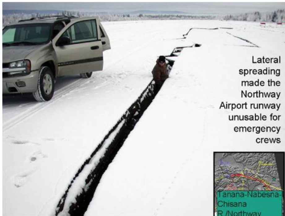
Figure 4-9 – Airport runway with lateral spreading, 2008 Denali Earthquake, Alaska
