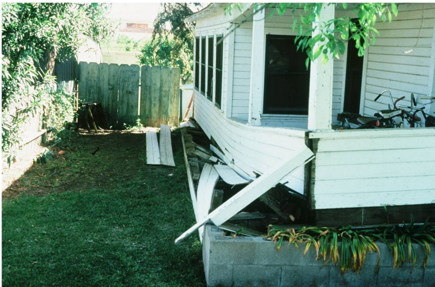
Figure 2-4 – House off of its foundation
