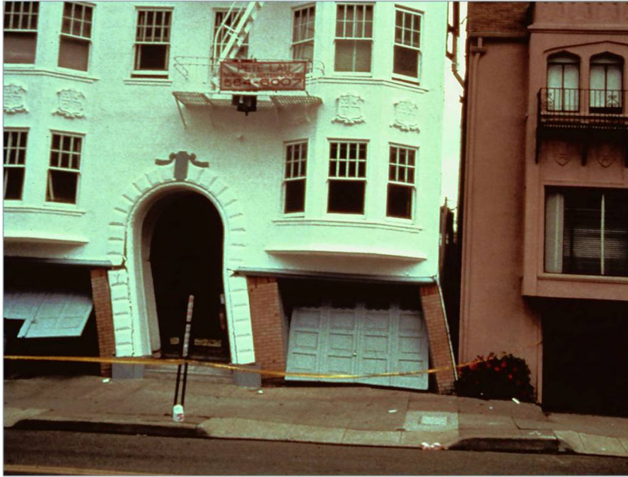
Figure 2-3 – Soft story failure, San Francisco, 1989 Loma Prieta Earthquake
