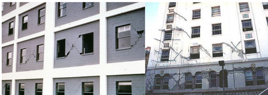
Figure 2-2 – Shear cracking
