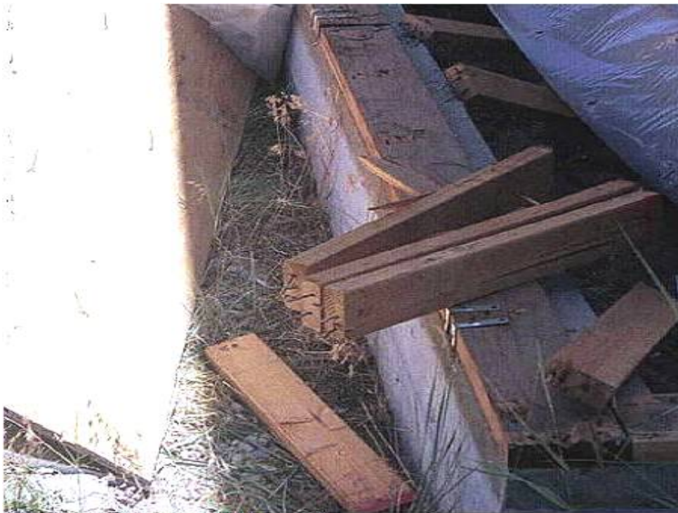
Figure 6-20 – House with cripple wall failure, 1992 Big Bear Earthquake
