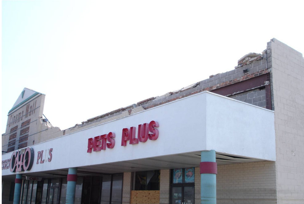
Figure 3-2 – Parapet blown off, 2005 Hurricane Katrina
