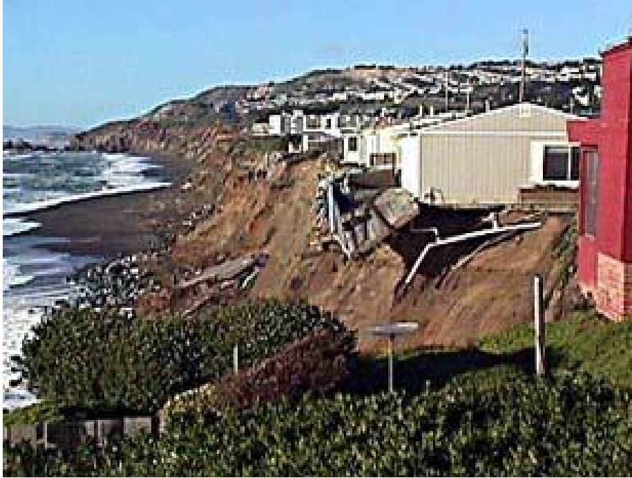
Figure 3-16 – Unsafe house due to cliff erosion, Pacifica, CA, 1998 El Nino Storms
