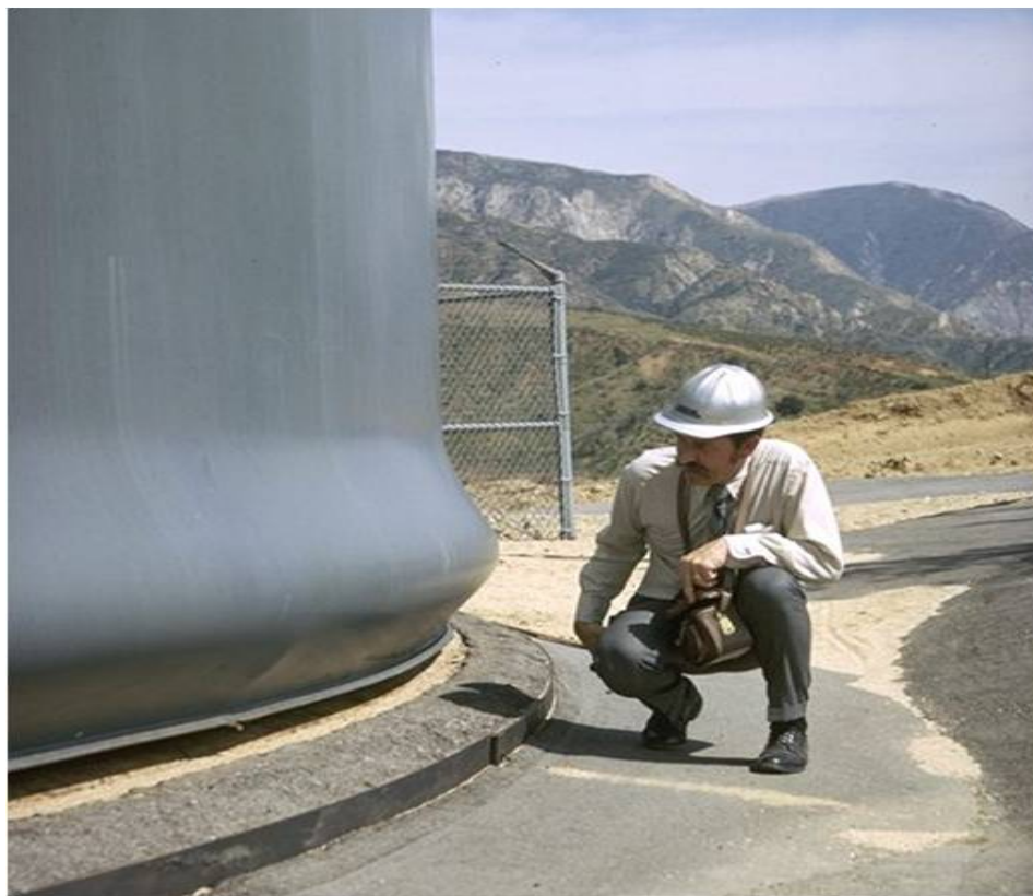
Figure 4-21 – Steel water tank with ‘elephant’s foot’ buckling
