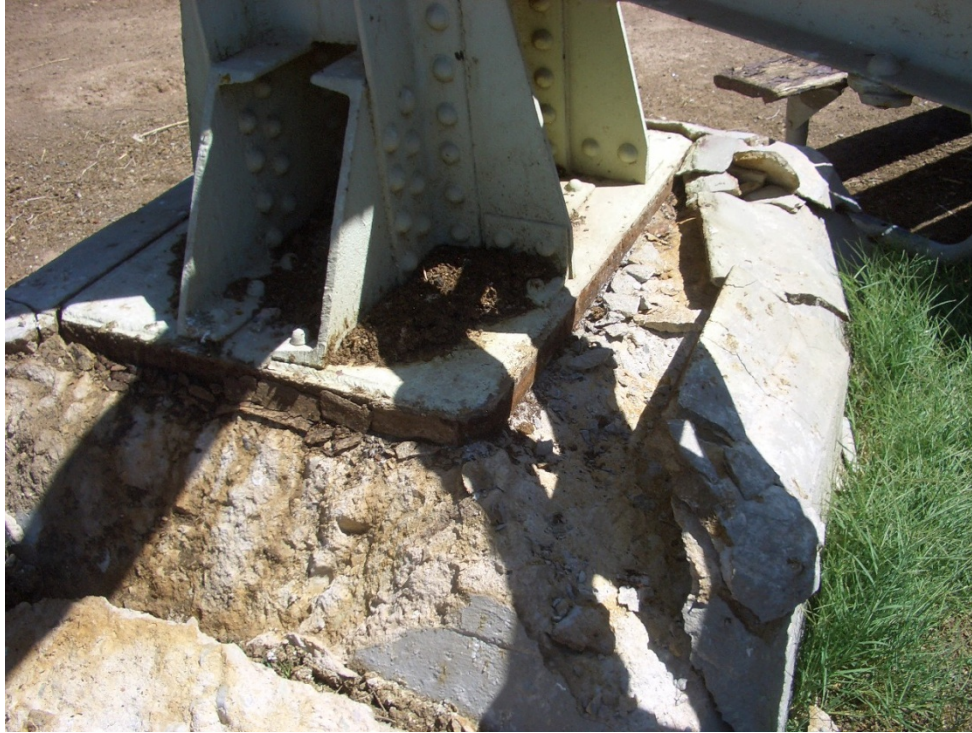
Figure 2-25 – Damage to water tower concrete footing
