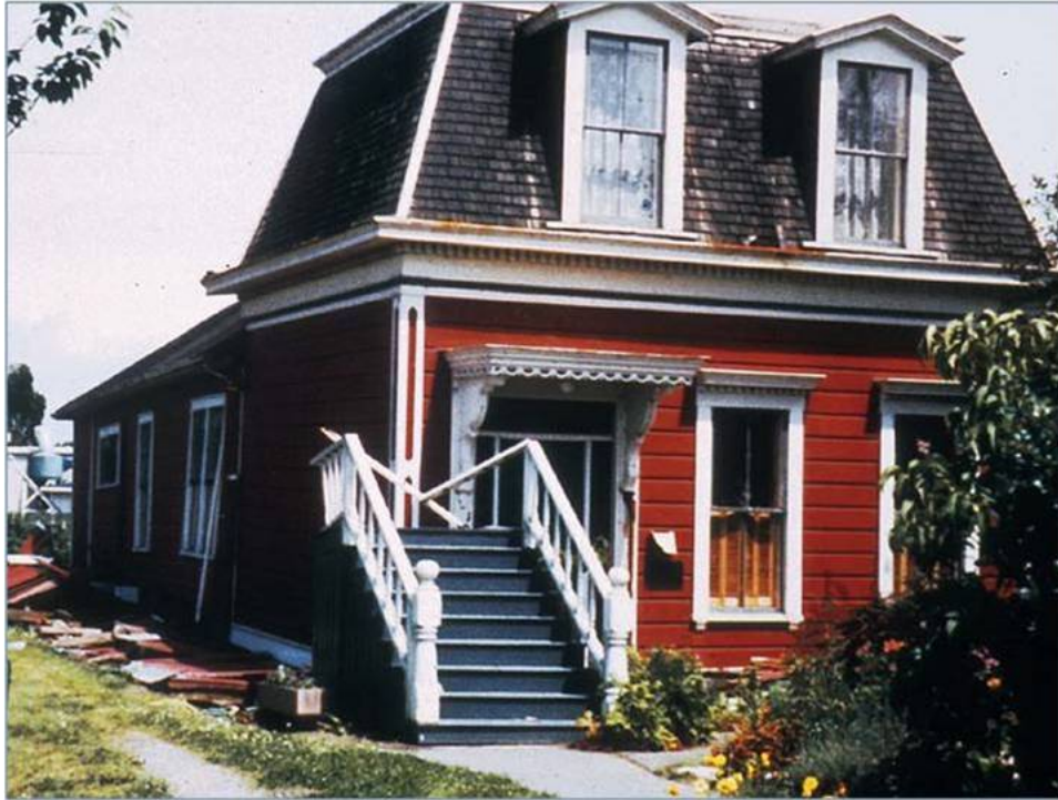
Figure 2-14 – Home collapsed on cripple walls, 1992 Humboldt Earthquake
