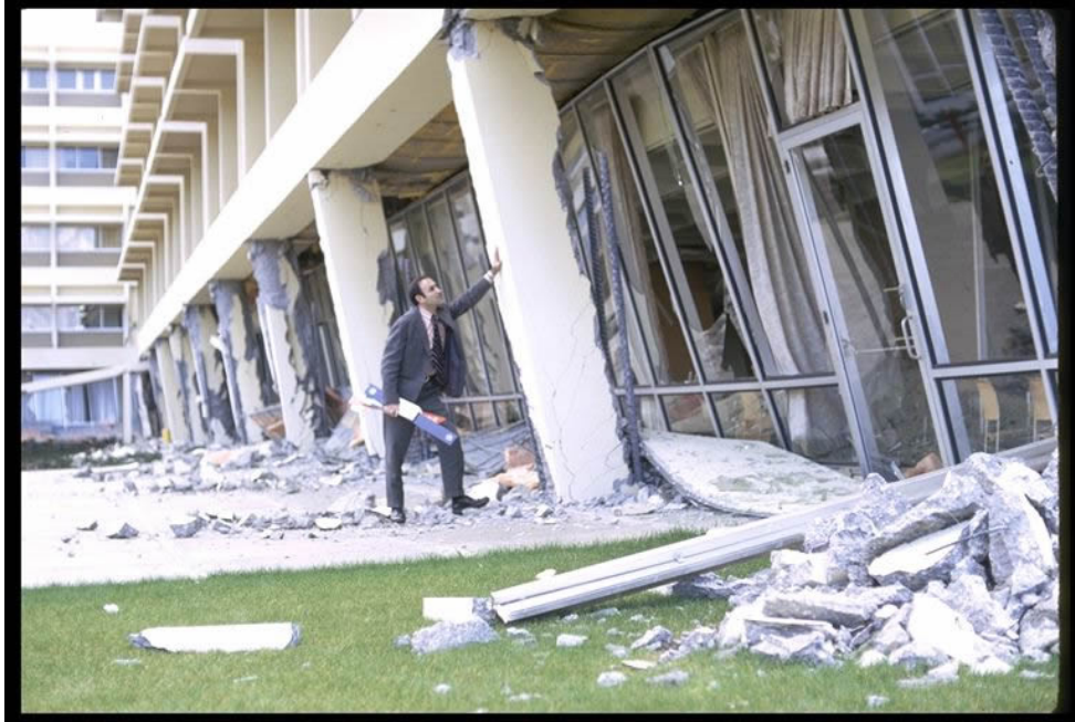
Figure 2-22 – Failure of concrete moment frame.
