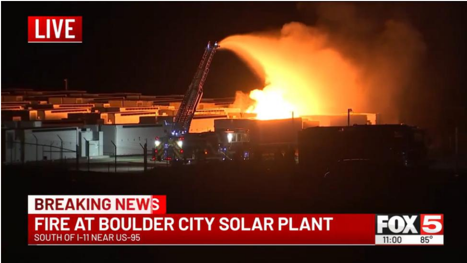
Fire (thermal) Hazard
