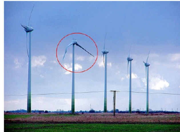
A damaged wind turbine at the centre of the Lincolnshire
