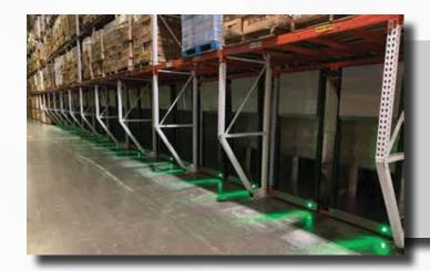
On-Demand freezing & tempering that works in existing racking to convert storage positions into blast positions overnight. Remote monitoring and control through wifi and integration into existing software through a standard API. Dedicated fan for each pallet ensures maximum performance and reliability.
