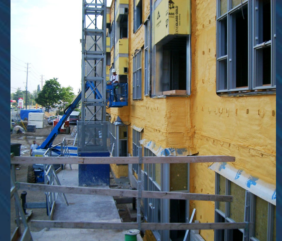
Building Enclosure Experience
