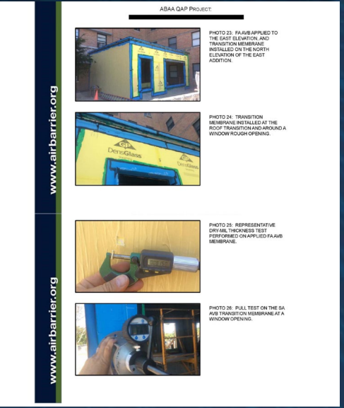
Photo log documenting installation
