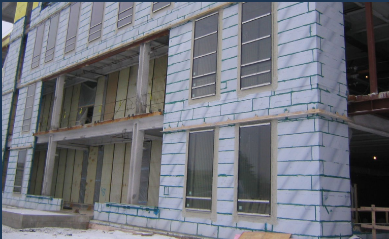
On-going Auditing of Quality Installations to Maintain Credential
