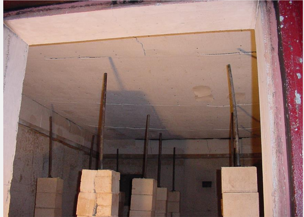
Exposed Side – After Test
