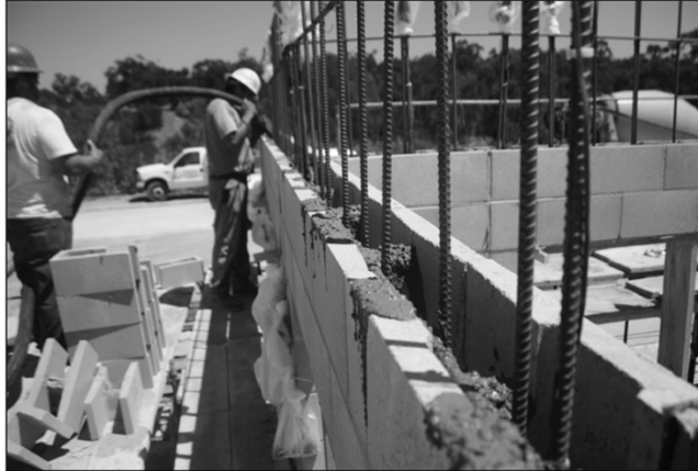
Grout flow is facilitated by open-end masonry units
